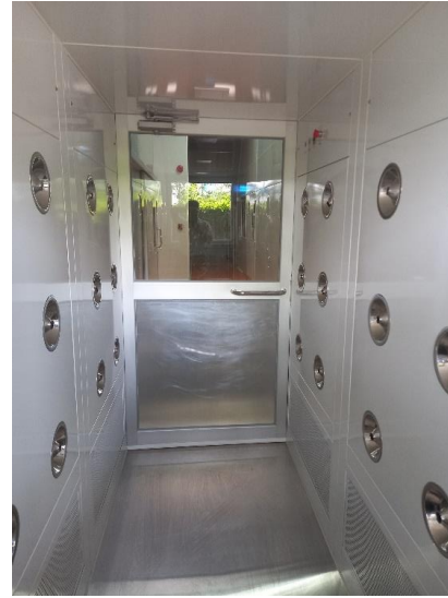
Air Shower System
